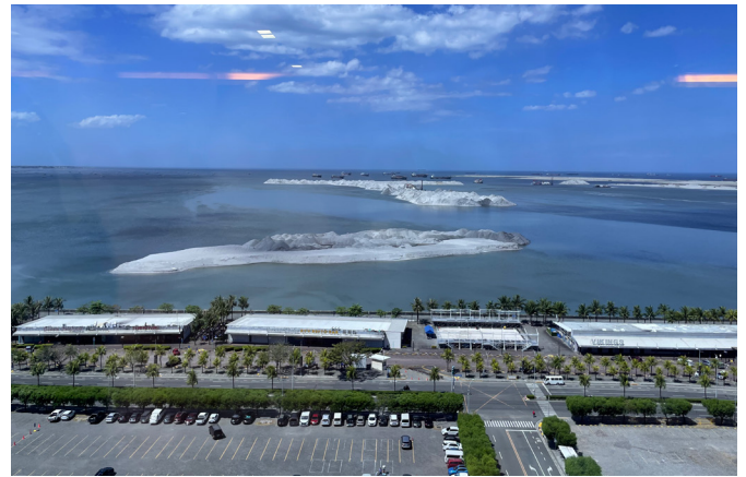
SM Pasay reclamation project, Manila.
