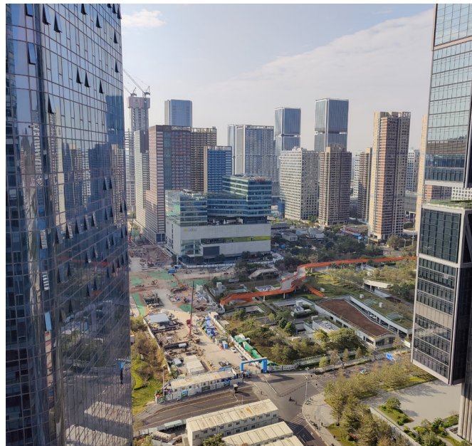
Buildings under construction on the outskirts of Shenzhen.
