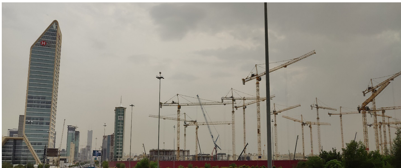
Riyadh under construction.
